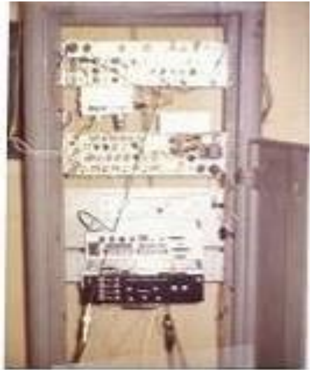
FIG 1: First Mt. Vernon Repeater, WA8ONN/R At the home of WA8ONN and WA8YRS
